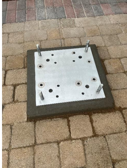
Piertech 3 Anchor Plate Shown Installed
