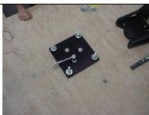
(3) Tighten Bolts. Tighten down anchor plate to deck.
