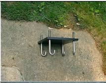
(5) Get Plate Ready. The cement mounting Pier-Tech Anchor Plate is shown here. The J bolts are secured to the bottom of the plate.
