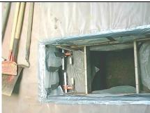
(3) Form top of hole. This is optional if you are making the top of the hole level with the ground and mandatory if you are going above the level of the ground with the cement.
