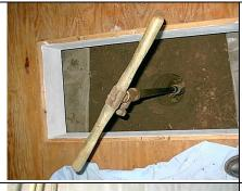
(1) Dig a Small Hole. Make a small hole approx. 6 inches in diameter x 36 inches deep. You can use a manual post hole digger for your local hardware store, or rent a power digger.
