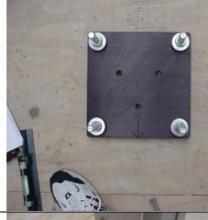
(2) Drill through Anchor Plate Holes. This marks the location for the bolts. \*With an Existing Cement Mounting, pound cement anchor studs through the Anchor Plate holes after drilling. Then tighten the cement anchor studs.
